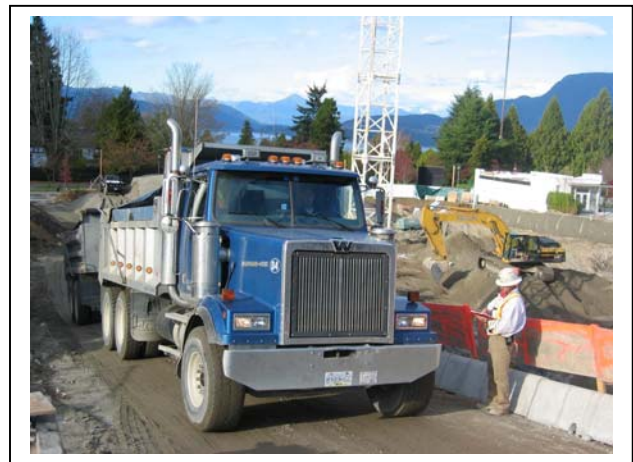
Truck Traffic Management Site Check
