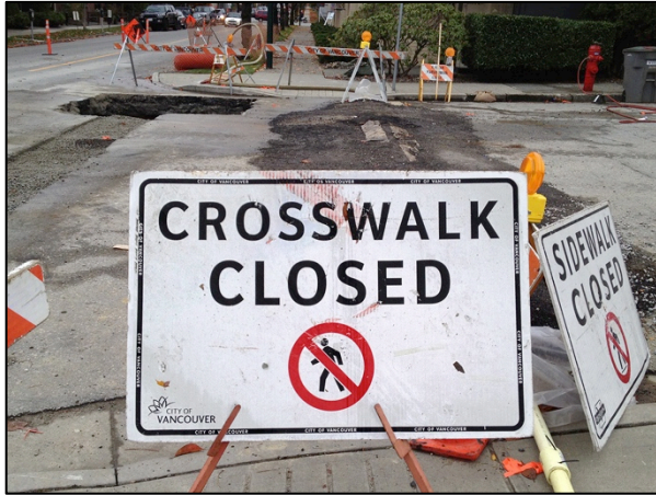
“Crosswalk closed” signs to be used at intersection or crossing. 900 x 600 mm.
