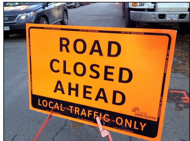
“Road closed ahead” sign to be used at intersection or decision point in advance of closure where motorists can detour around closure. 900 x 600 mm.
