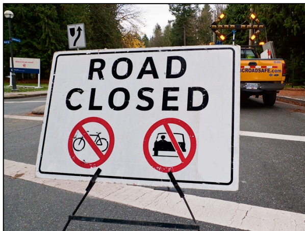
“Road closed” sign to be used at closure. 900 x 600 mm.
