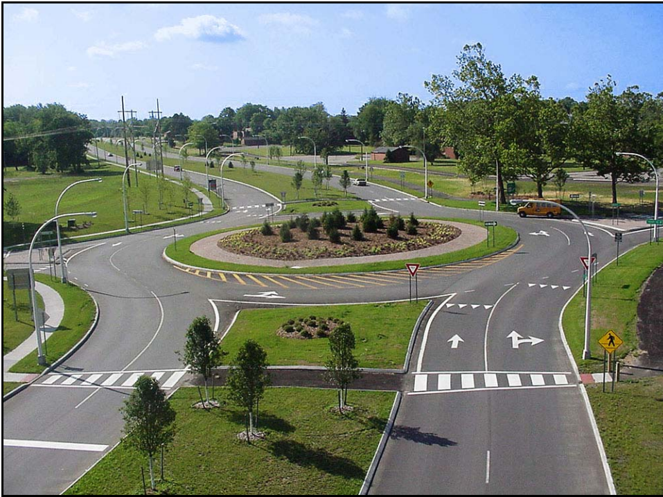
Source: New York State Department of Transportation
