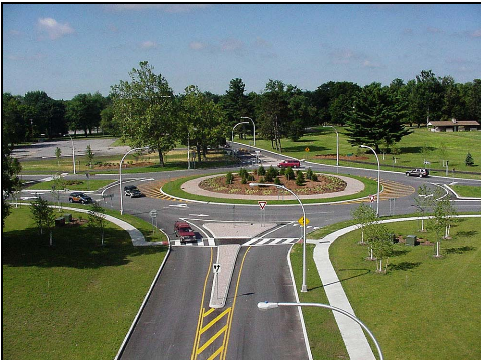
Source: New York State Department of Transportation
