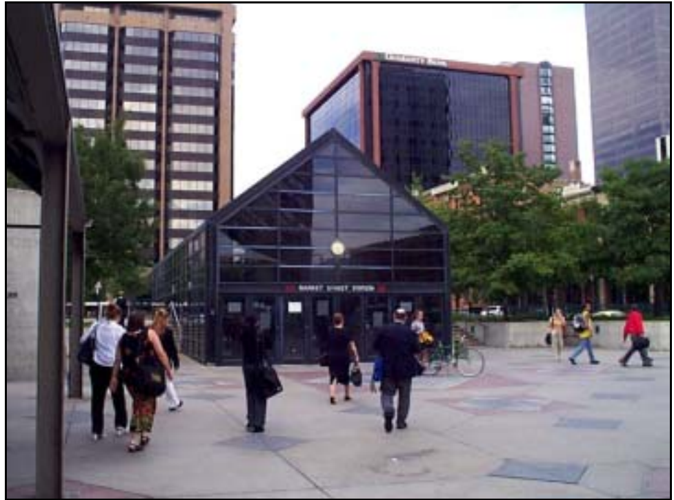
Figure 6.8: Below-Grade Bus Transit Station – Denver, Colorado
