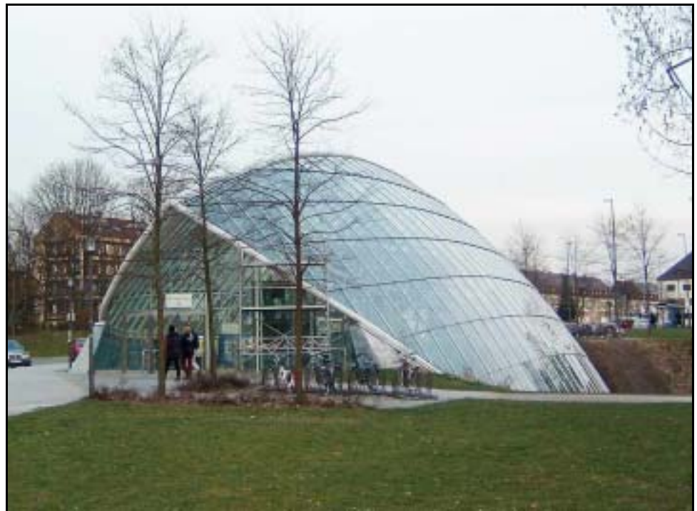
Figure 6.15: Below-Grade Transit Station – Munich, Germany
