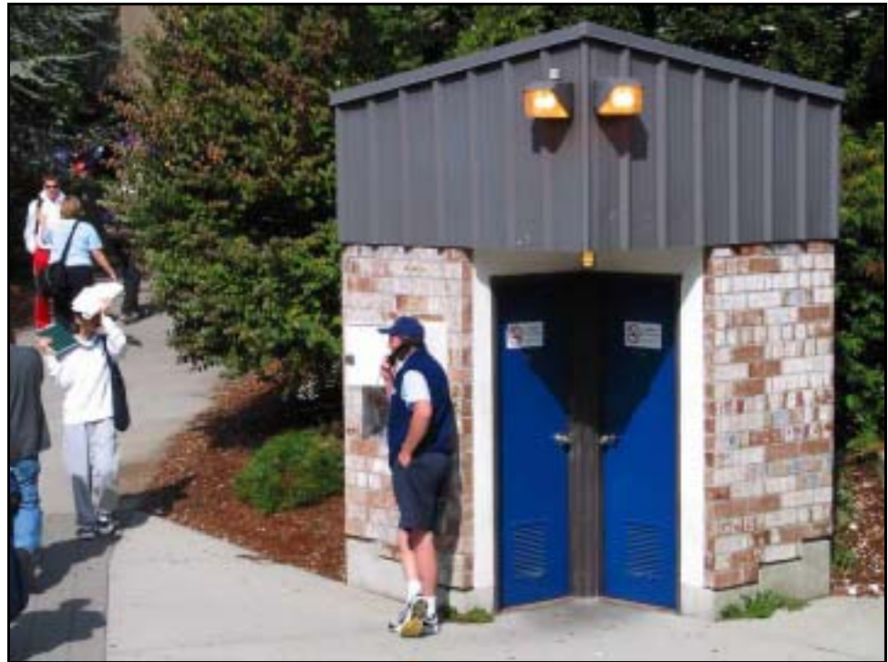
Figure 2.4: Drivers' Facilities at Bus Loop
