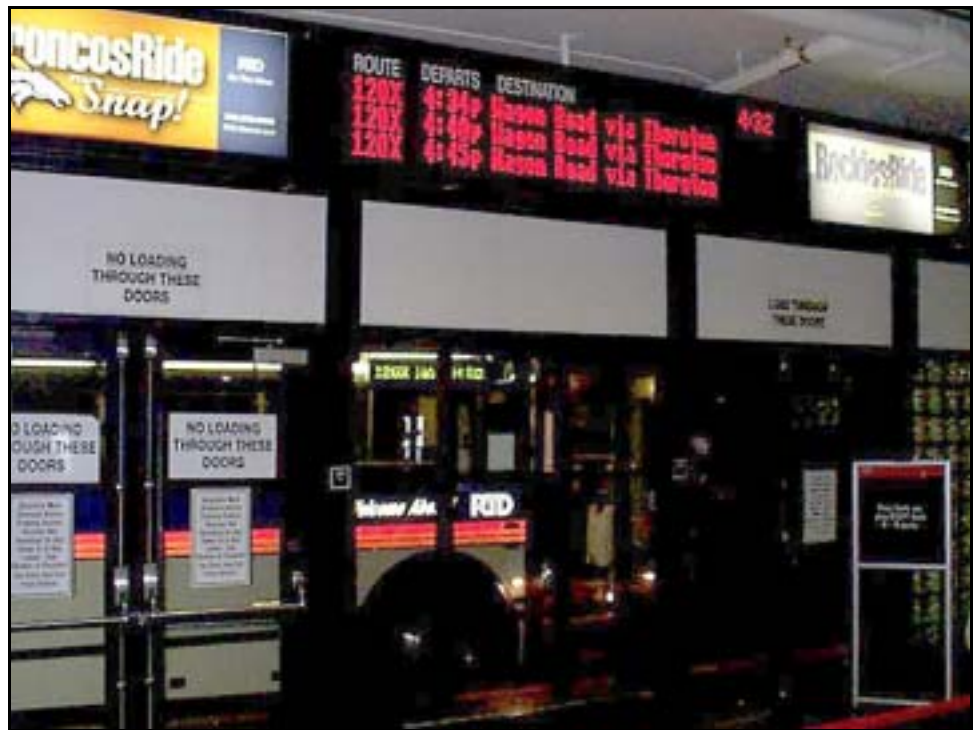
Figure 6.9: Below-Grade Bus Transit Station – Denver, Colorado
